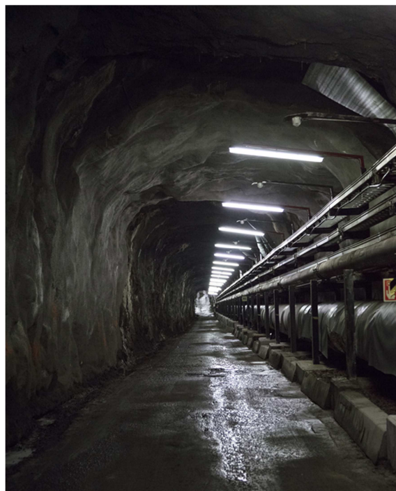
Figure 3: Mustikkamaa rock cavern in Helsinki. Photo: Helen Ltd.
