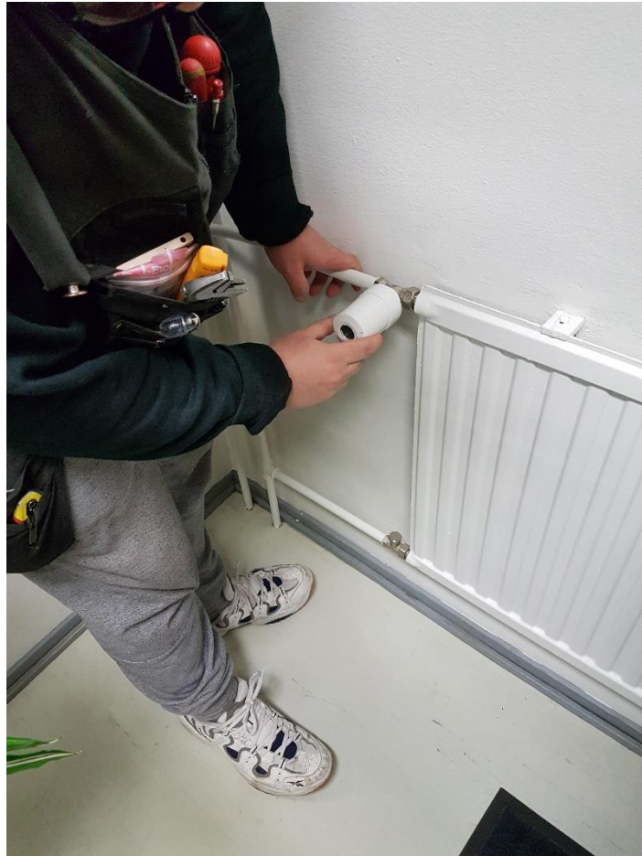
Figure 6: Installing smart thermostat in the office in Helsingin Merihaka Oy. The thermostat was installed as an example and a tool for advising the residents
