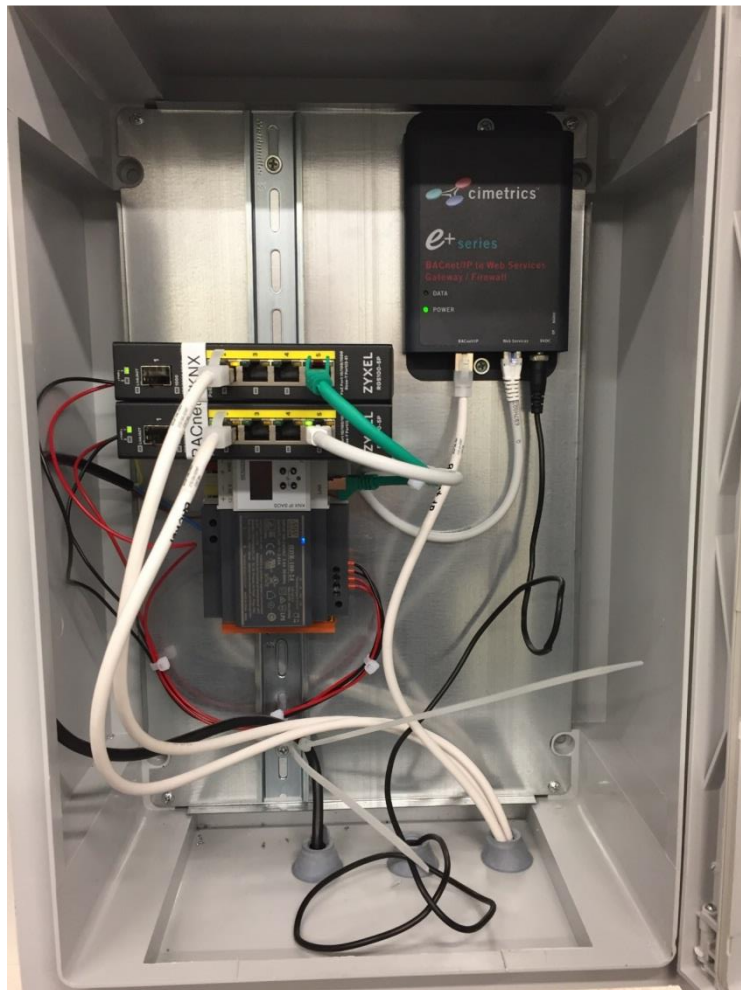
Figure 8: Viikki Building Automation Gateways
