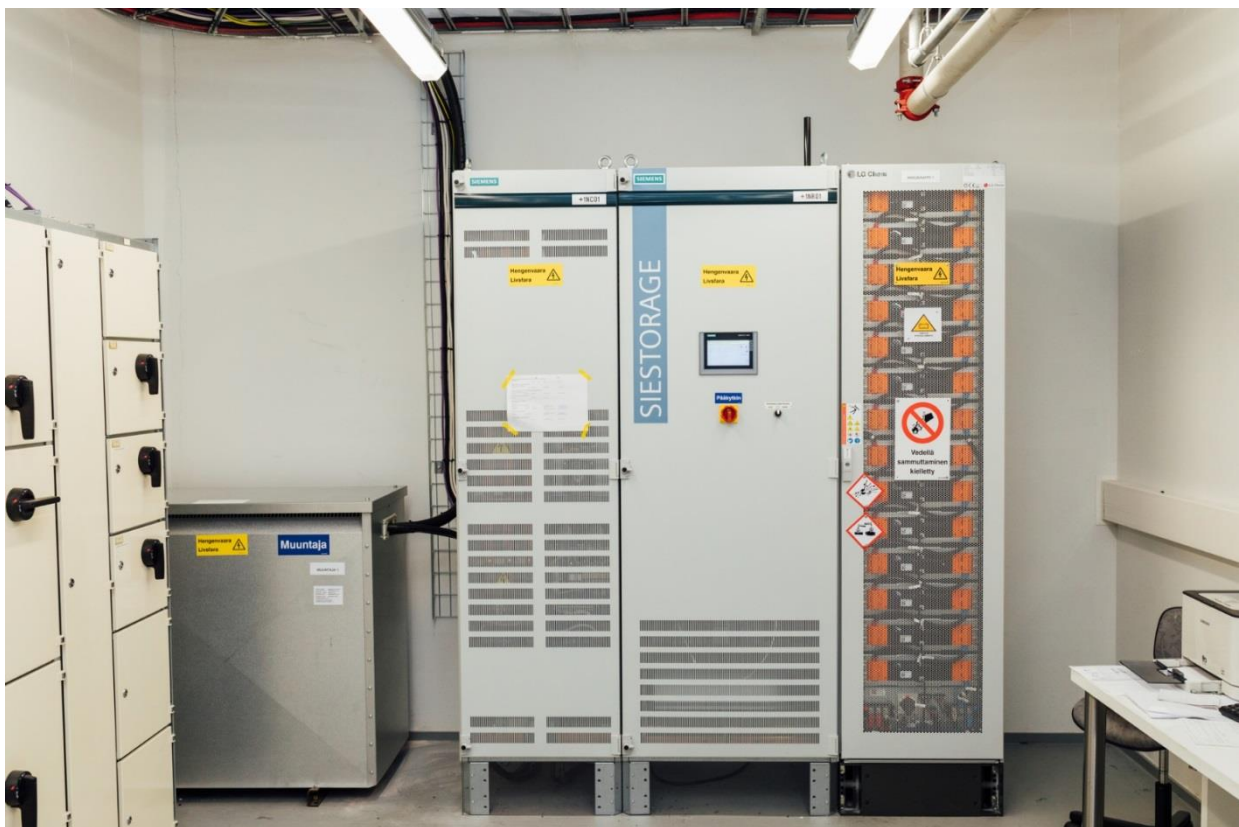
Figure 13: The battery energy storage at Viikki Environment House used to optimize the building's own energy production and consumption (Helen, 2017, photo by Niklas Sandström)
