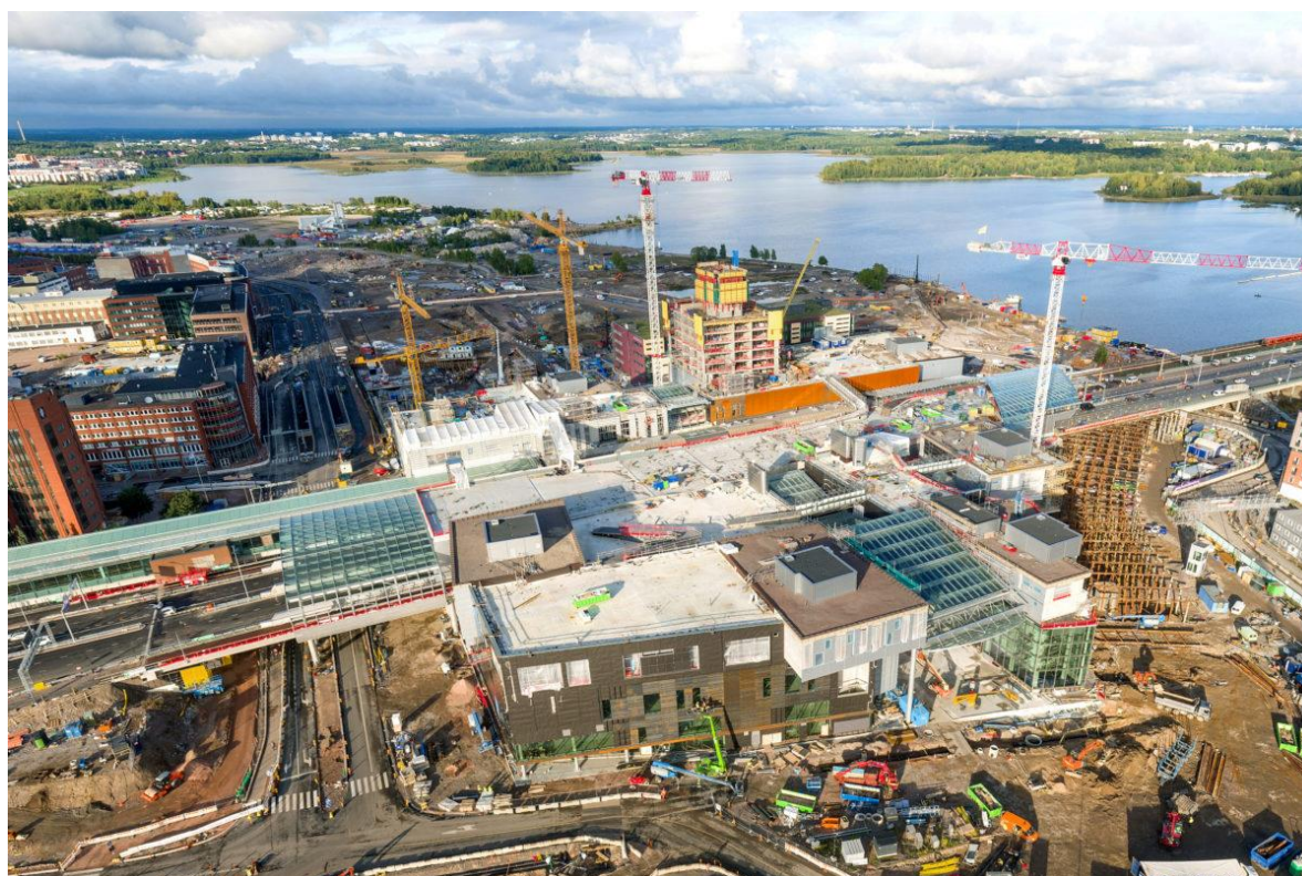
Figure 6: Kalasatama construction site in 2017 (figure from HEL)
