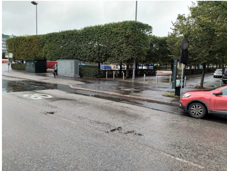
Figure 5: Charger electrical cabinet. The charging mast is behind the trees at 50 m distance
