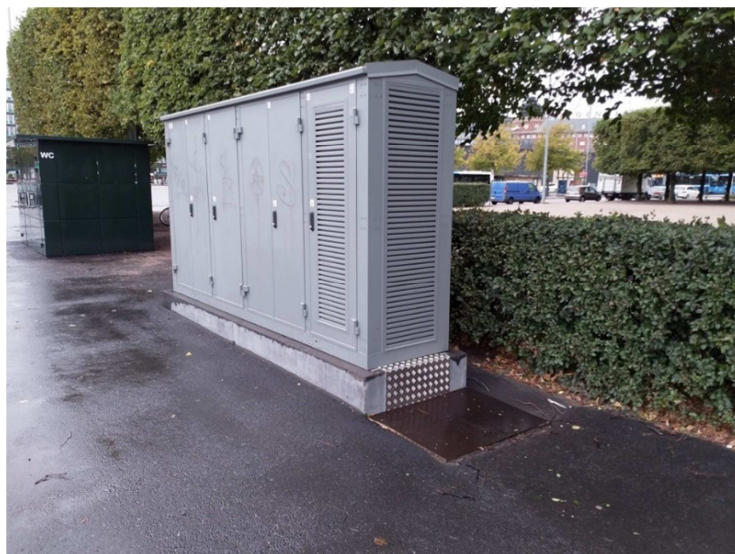
Figure 6: Reserved spot for installing the cabling for the additional electrical cabinet
