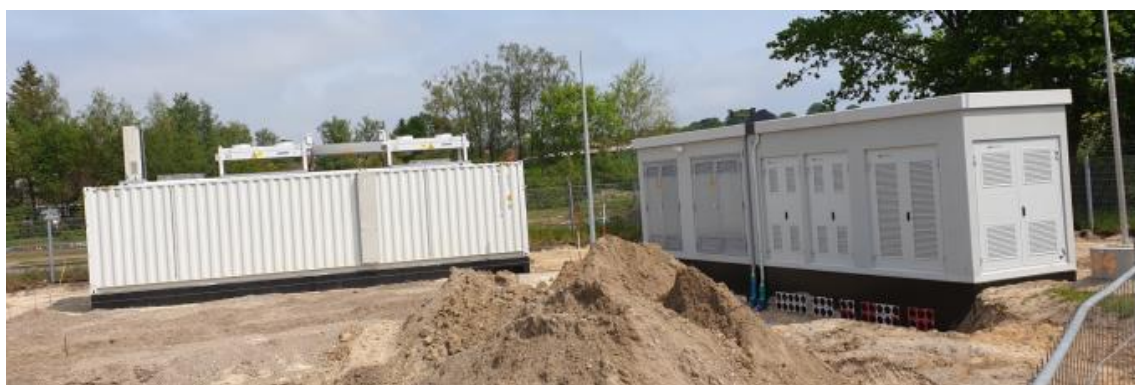
Figure 7: Battery storage container on the left, combined transformer and inverter station on the right [source: VHH]
