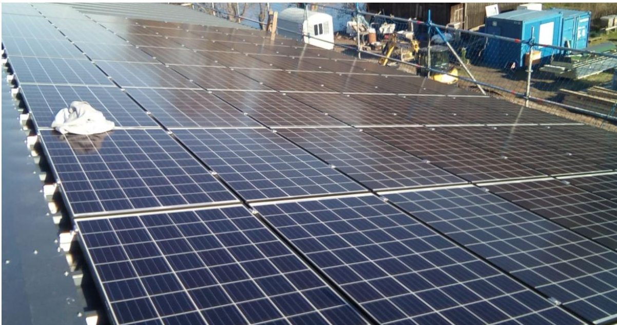
Figure 5-7: PV-plant Ochsenwerder just before completion, Foto Clen Solar
