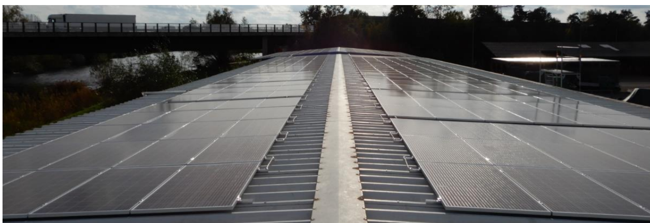
Figure 5-6: PV-modules on the roof Kampweg 4, source: ENH
