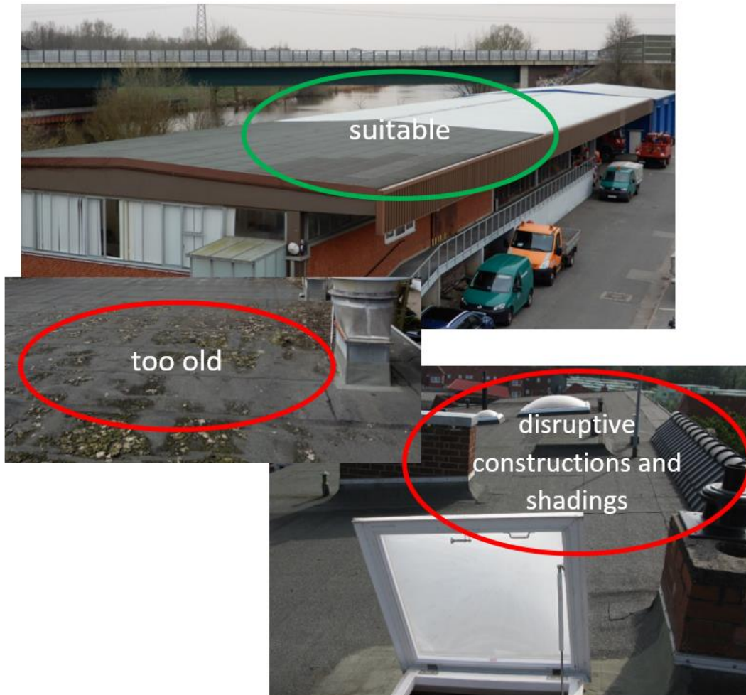
Figure 5-1: Suitable and unfitted roof tops – source ENH
