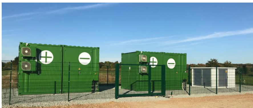
Figure 4-2: battery storage at the wind farm curslack, source: HAW own
