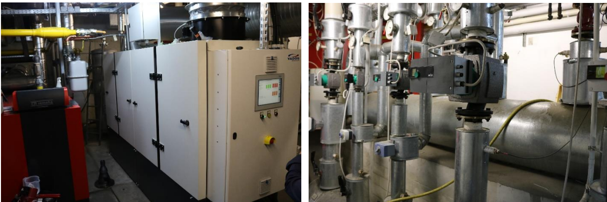
Figure 6 New heating central at heating island H4 Hotel (konsalt GmbH).
