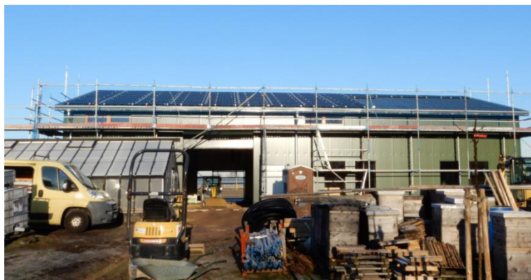
Figure 26: The Ochsenwerder beekeeping with the PV plant under construction (Source ENH).
