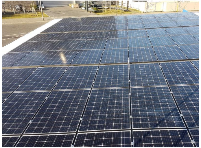
Figure 23: The PV-plant of GALAB (source ENH).
