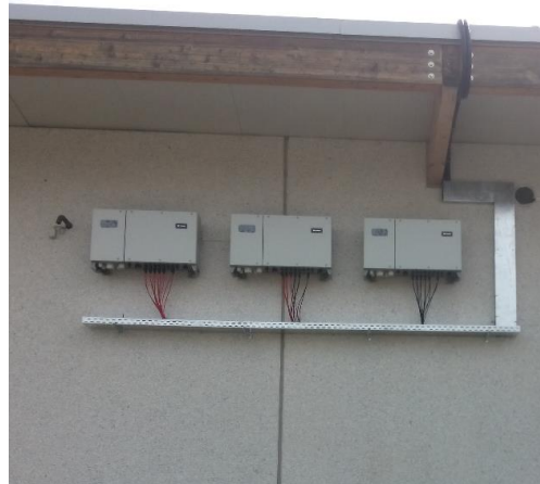
Figure 25: The inverters of the PV system on the outside wall (source ENH).
