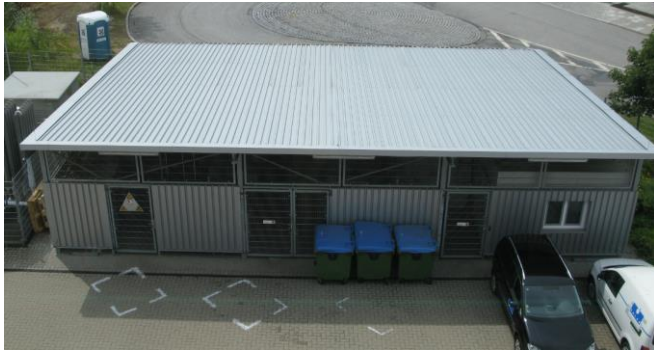
Figure 22: The open storage building of GALAB, on which the PV system will be installed (source ENH).
