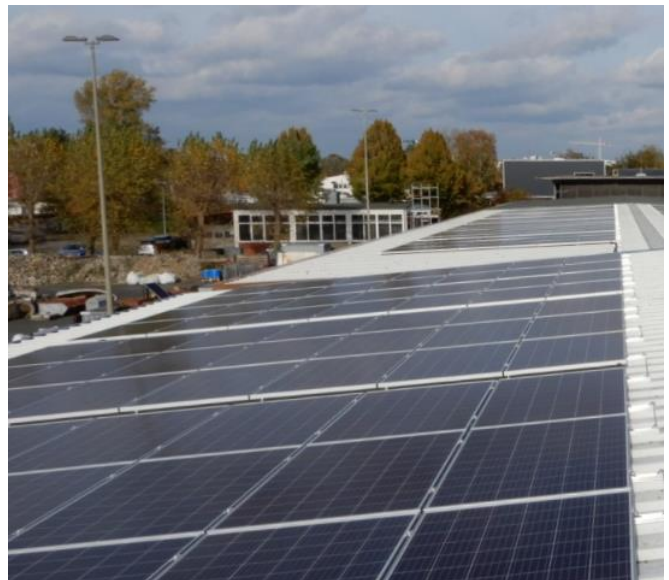
Figure 16: View over the finished PV plant Kampweg (source ENH)
