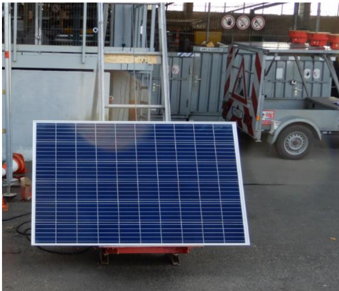
Figure 15: Construction of the plant: Module on a roofer's elevator (source ENH)
