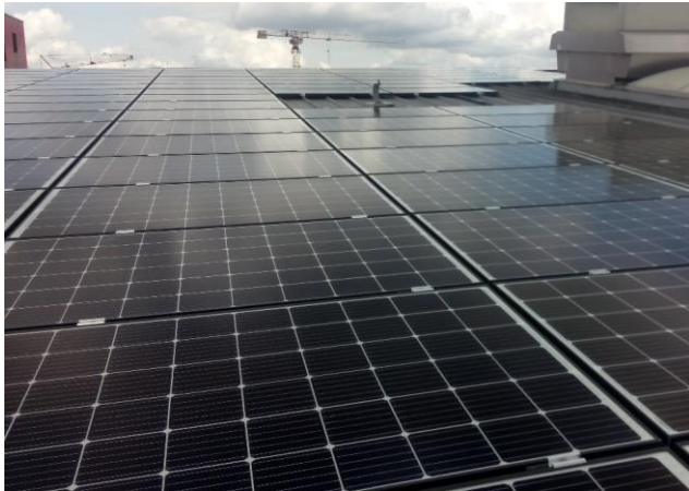
Figure 24: The PV system on the roof of the organic bakery (Source ENH).
