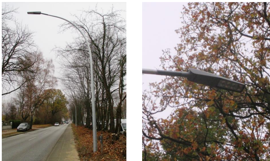
Figure 6: The retrofitted lamppost with LED lights (own source)
