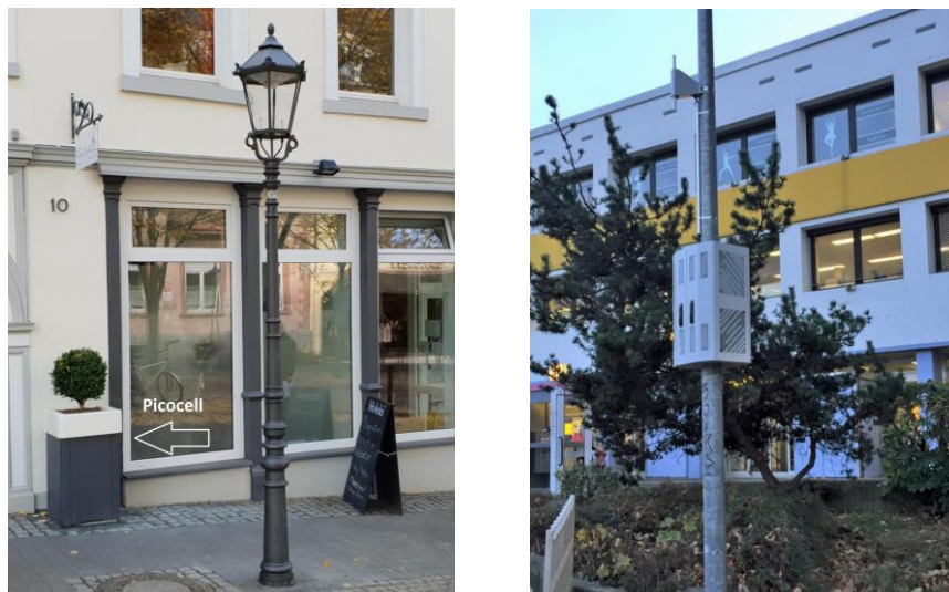
Figure 7: Two examples to implement picocells: at the left the cell is hidden as a flower pot, at the right the cell is directly mounted at a lamp pole (source DT)
