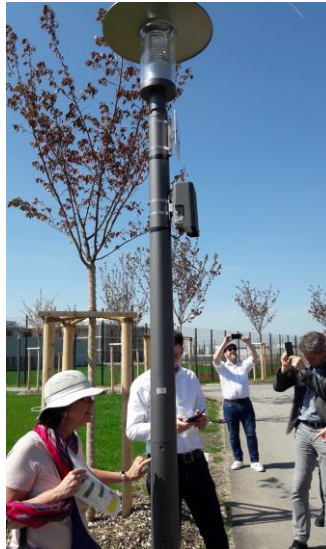
Figure 3: Smart street light in Munich (own source)
