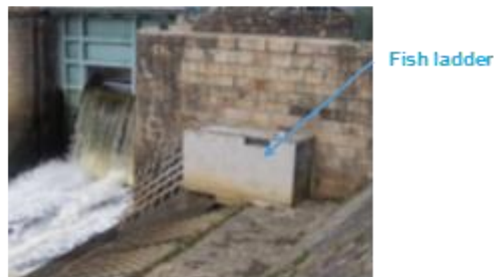
Figure 40: Example of fish ladder to ensure the ecological continuity
