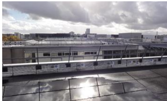
Figure 30: Roof of CIC building
