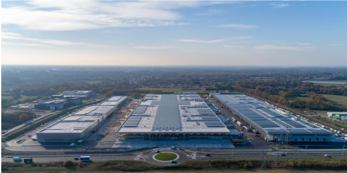
Figure 2: The MIN buildings and the solar plants on the roofs (source: Nantes Metropole)
