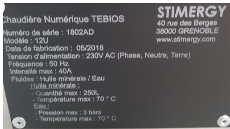
Figure 8: Technical description of the digital boiler in Oiseau des Iles
