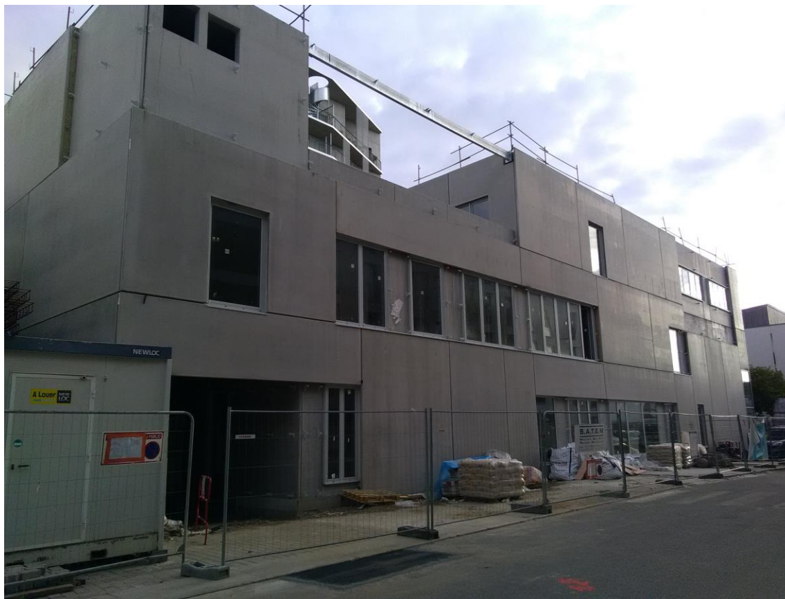
Figure 12: The building under construction (picture by Nantes Métropole)
