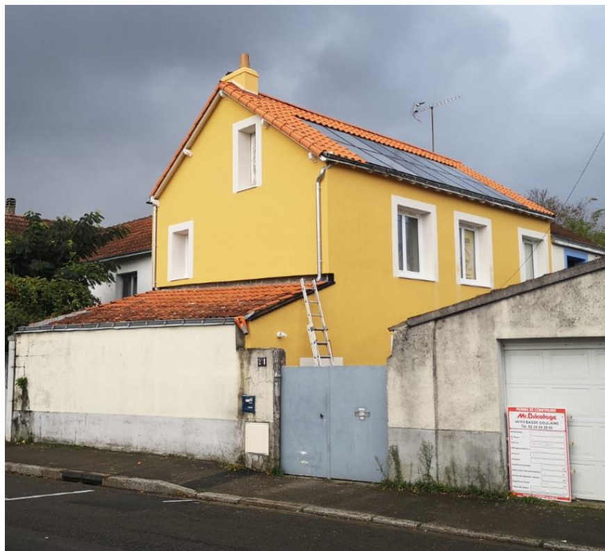
Figure 14: The house after the renovation works
