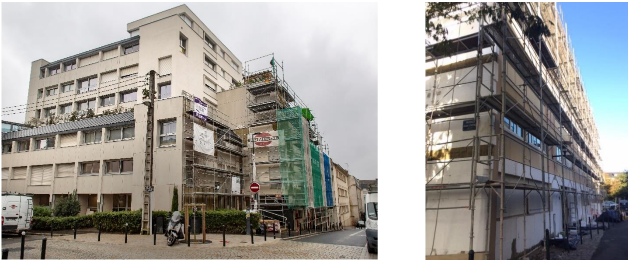
Figure 33: Massillon facade during retrofitting works
