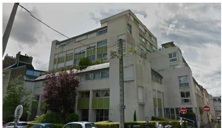
Figure 31: Massillon facade before retrofitting works
