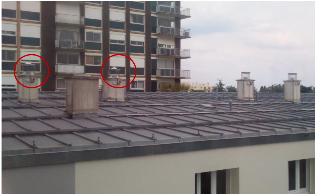
Figure 41: Fan support of Nantes-Paris hybrid ventilation using existing duct
