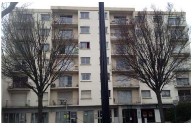
Figure 27: Le Strogoff before retrofitting work
