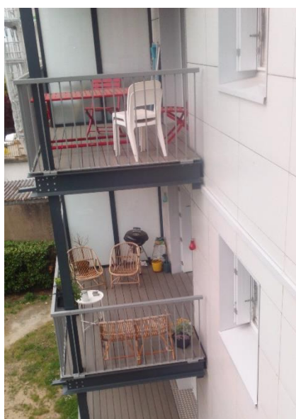
Figure 34: Disconnected balconies of Val de Loire after retrofitting
