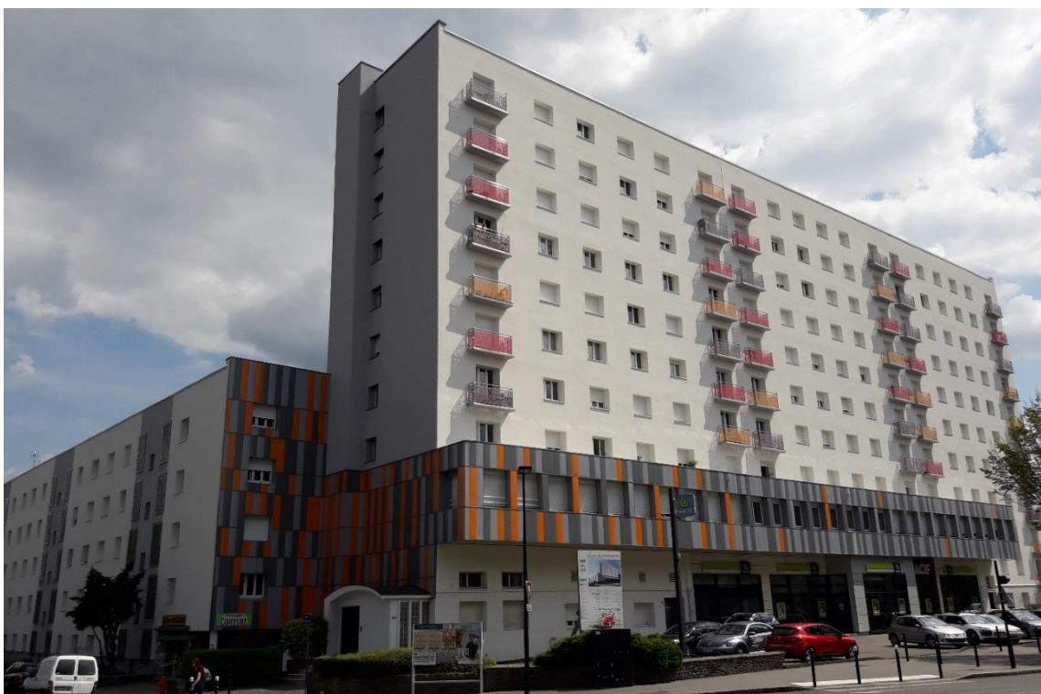
Figure 22: Nantes Paris after retrofitting works
