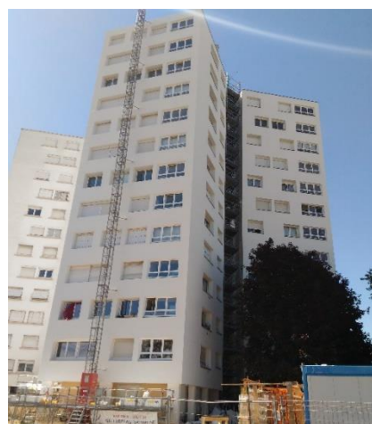
Figure 24: Benoni-Goullin during retrofitting // Architect: Mervane architectes
