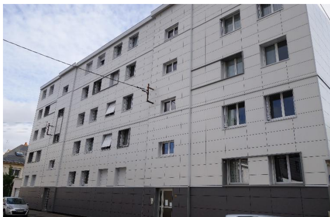
Figure 28: North West Facade of Val de Loire after retrofitting
