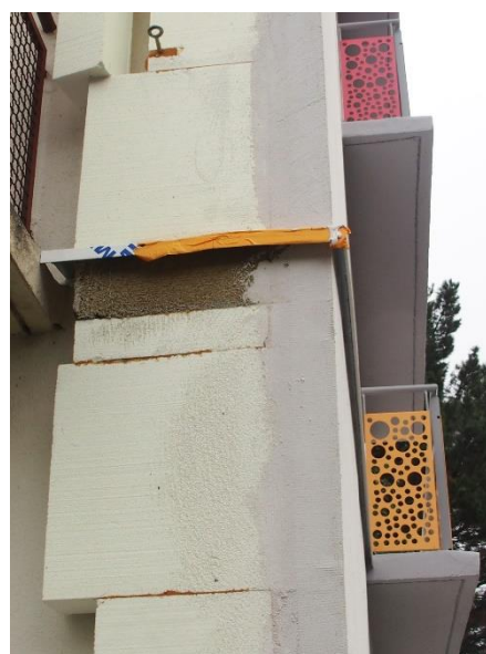
Figure 35: Nantes-Paris - external insulation during works
