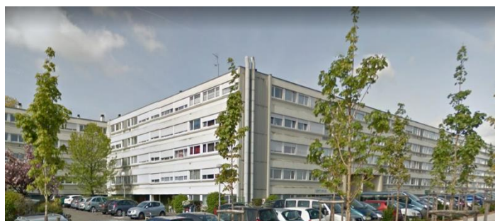
Figure 12: Le Parc building
