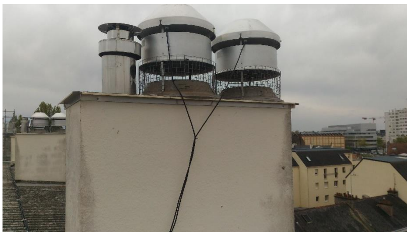
Figure 40: Fan support of Val de Loire hybrid ventilation
