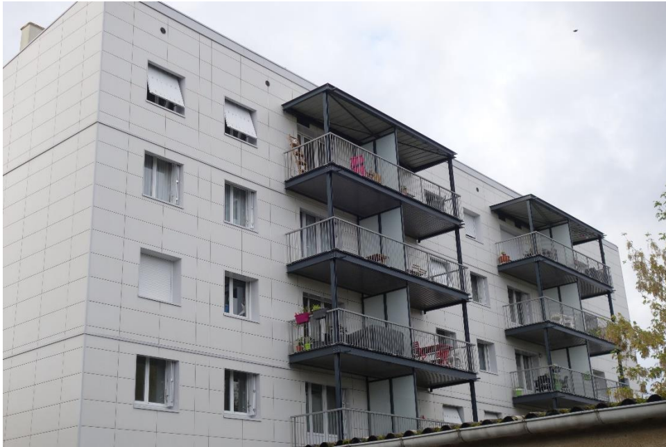
Figure 30: South East Facade of Val de Loire after retrofitting Works
