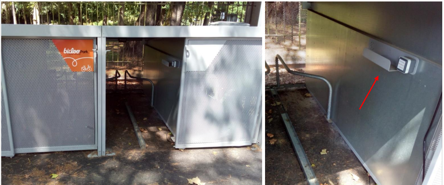
Figure 31: Individual boxes with electric socket inside
