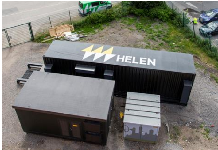
Figure 18: Battery Energy Storage System (photo: Helen Ltd.)
