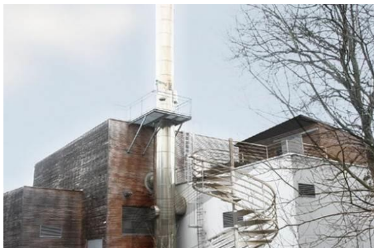
Figure 5: Chantrerie biomass boiler plant
