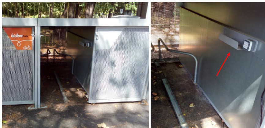
Figure 31: Individual boxes with electric socket inside
