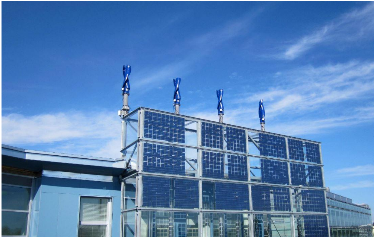
Figure 14. Small vertical axis wind turbines at Viikki office building (figure from HEL)
