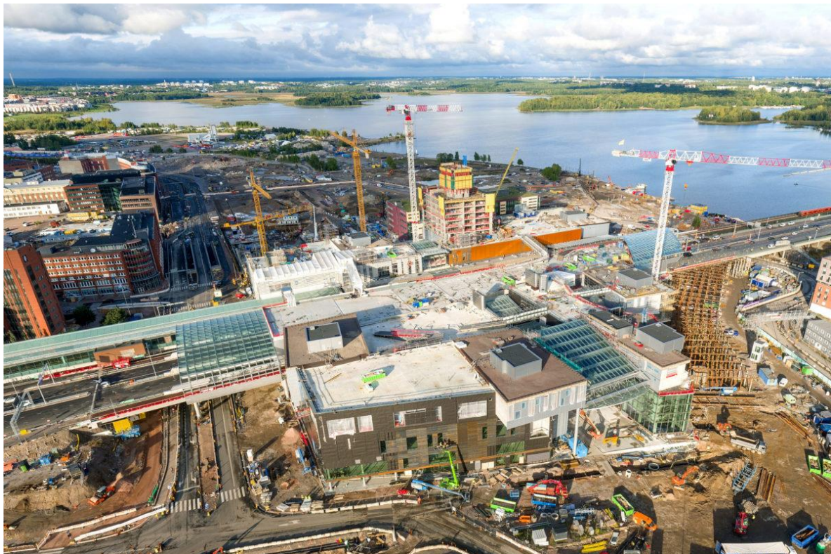
Figure 6. Kalasatama construction site in 2017 (figure from HEL)
