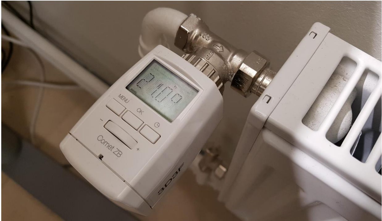
Figure 15. Smart thermostat at Viikki office building (figure by HEL)
