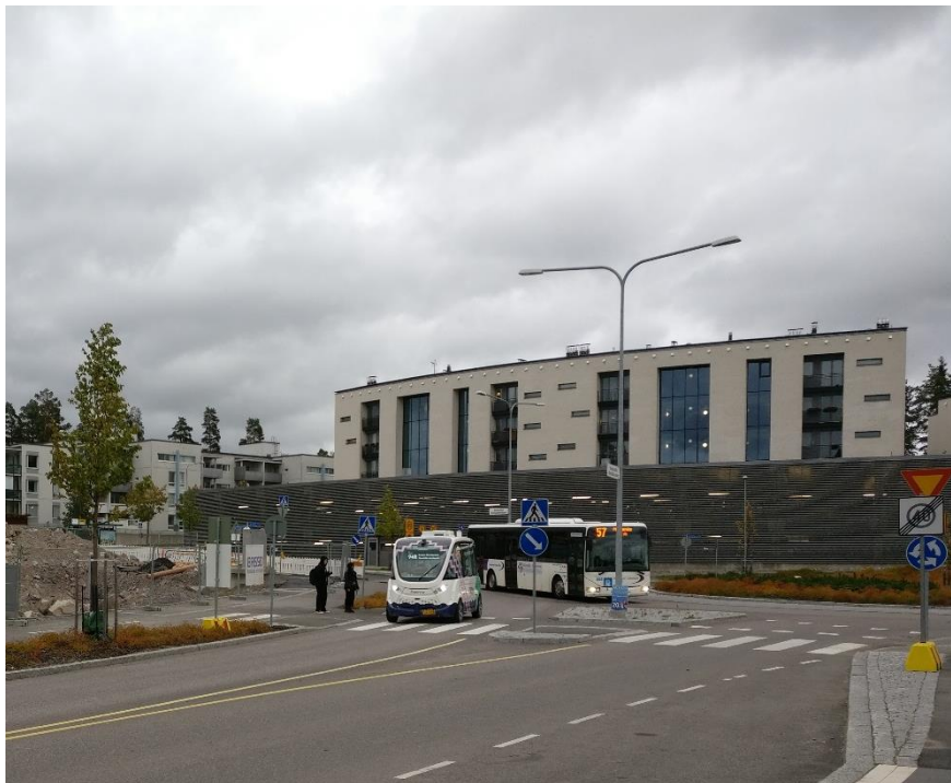
Figure 14: Roundabout at Kivikonlaita stop [Rutanen 2018].
