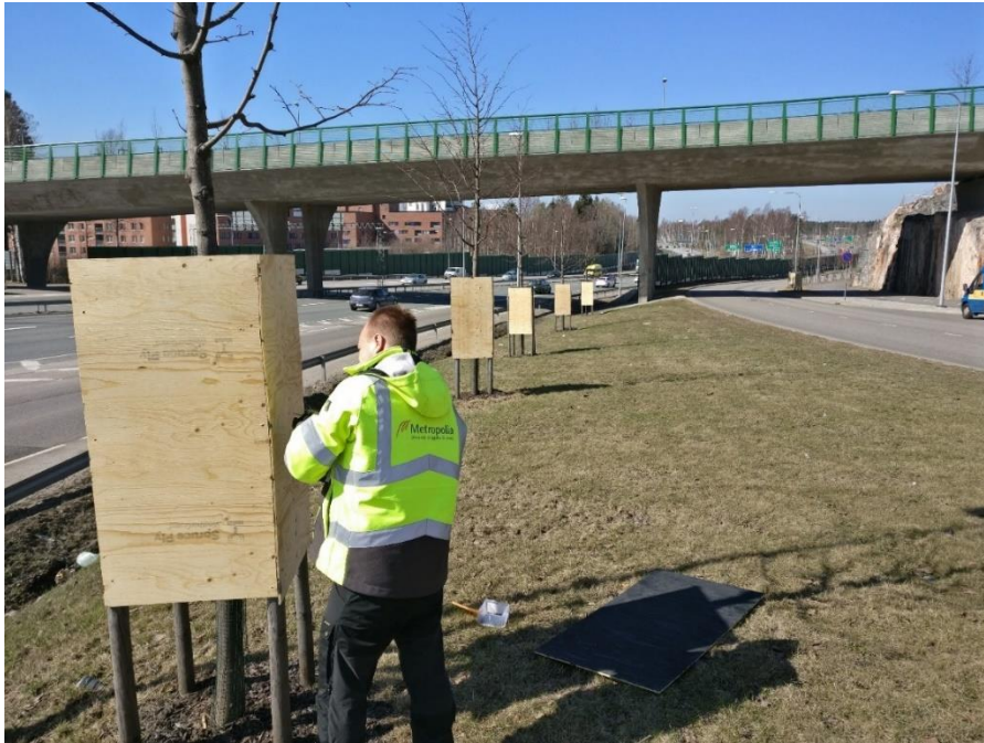
Figure 20: Installation of wooden constructs to frames of growing trees near the bridge at the Kivikonlaita road [Rutanen 2018].
