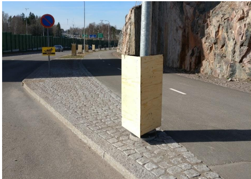
Figure 21: Wooden construct around a lamppost near the bridge at Kivikonlaita road [Rutanen 2018].
