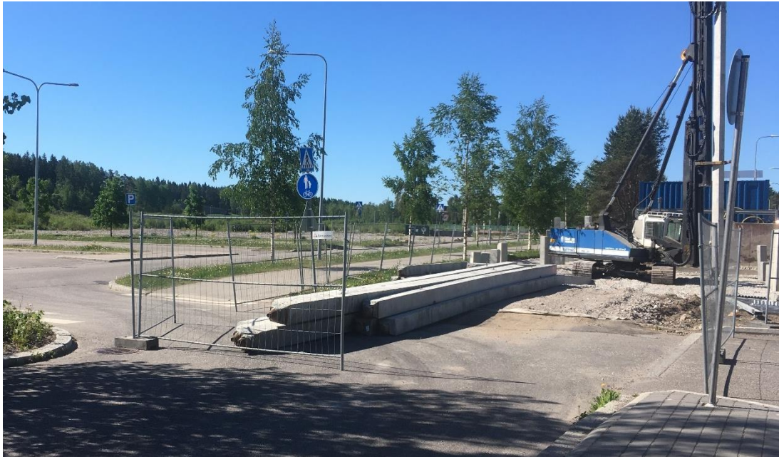
Figure 38: Construction supplies on the robot bus's path in Kivikko [Rutanen 2018].
