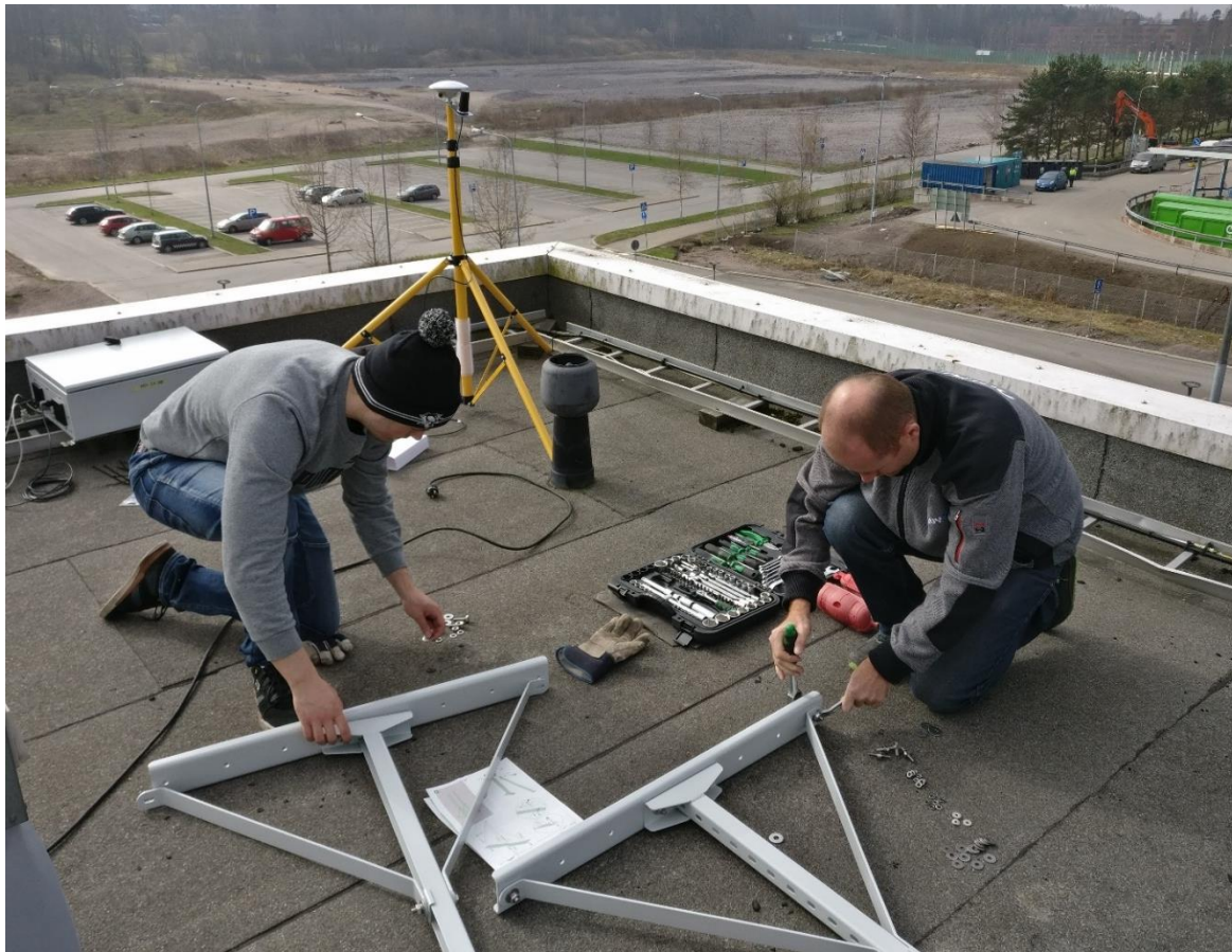
Figure 25: Fixed RTK GNSS reference station installation on the roof of the Kivikko Skiing hall [Rutanen 2018].
