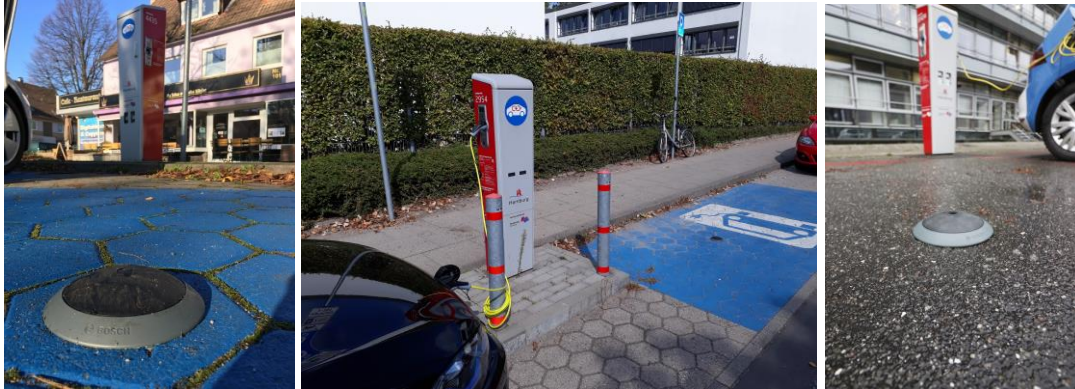
Figure 10: Selected ground sensors in practical test (Source: SNH'own photo)
