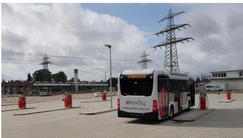
Figure 8: double charging points at VHH depot Bergedorf with 12m EvoBus connected for a first charge test [source: VHH]
