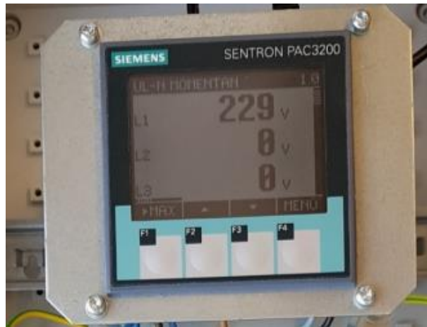
Figure 29: Multifunctional meter “Sentron PAC 3200” [Source: HAW]
