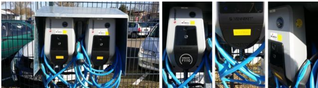
Figure 24: Visualisation of the hardware installation at the demonstration site Kampweg (Source: SNH)
