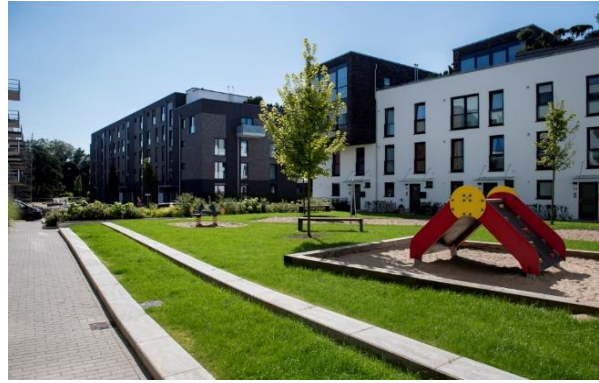
Figure 9: Picture of the new construction area “Glasbläserhöfe”(konsalt, 2017, own source)
