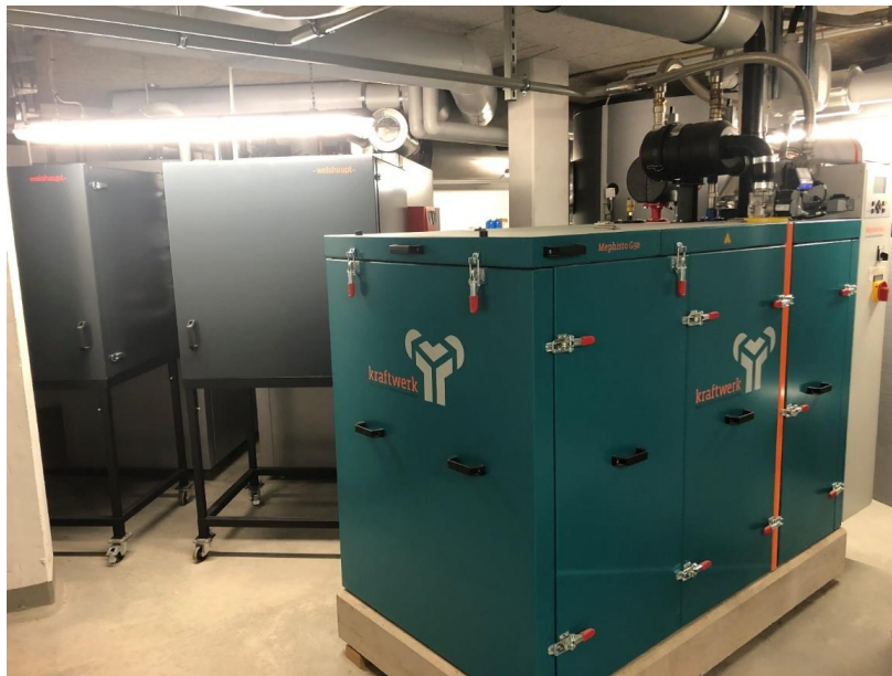
Figure 13: Picture of the used CHP (enercity, 2019, own source)
