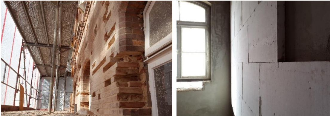
Figure 49: Retrofitting of the brick facade with calcium silicate interior insulation (konsalt, based on pictures of Metropol Grund, 2017)
