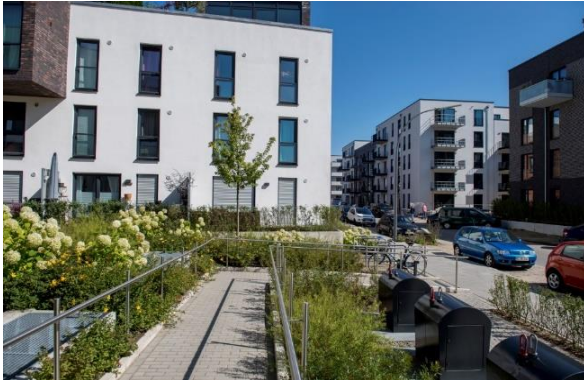
Figure 8: Picture of the new construction area “Glasbläserhöfe” (konsalt, 2017, own source)
