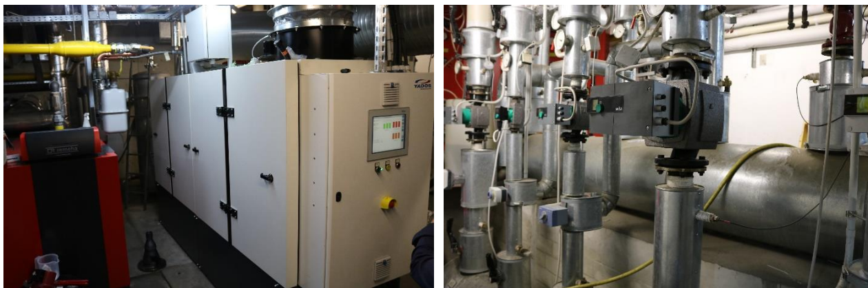
Figure 47: The new CHP plant in the H4 Hotel which supply heat to additional 50 apartments in the neighbour block (konsalt, own source, 2019)
