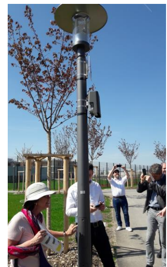
Figure 3: Smart street light in Munich (own source)
