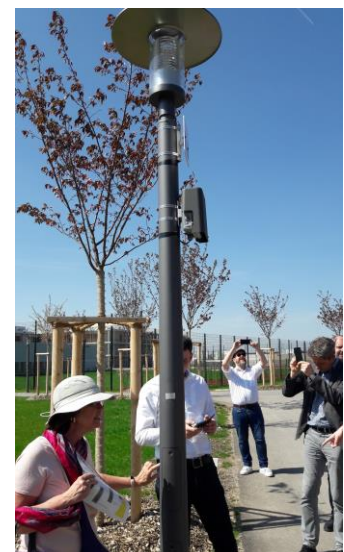
Figure 3: Smart street light in Munich (own source)
