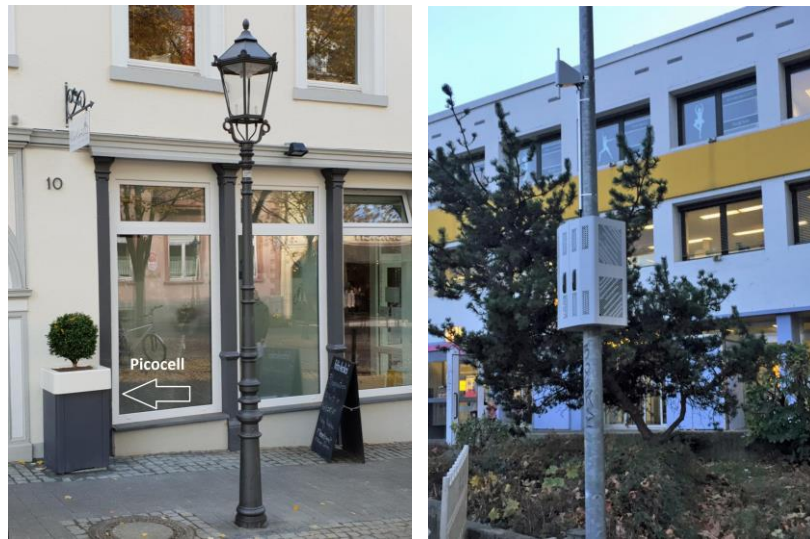
Figure 7: Two examples to implement picocells: at the left the cell is hidden as a flower pot, at the right the cell is directly mounted at a lamp pole (source DT)
