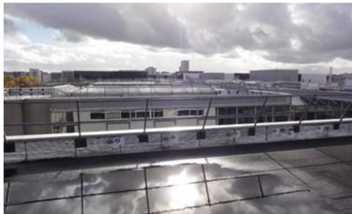
Figure 30: Roof of CIC building
