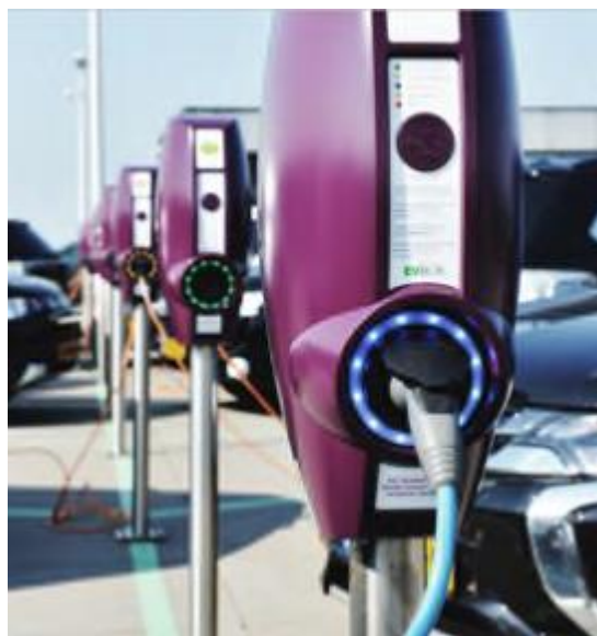
Figure 33: EV charging station
