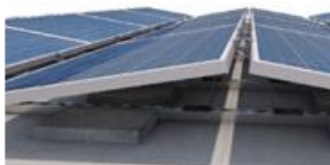
Figure 31: Example of PV panels for CIC building
