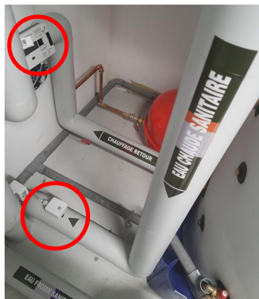
Figure 19: Temperature sensors and calorimeter in “Oiseau des Iles” building
