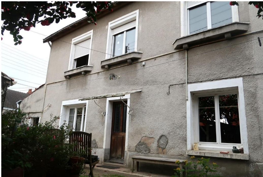
Figure 10: Picture of the house before works
