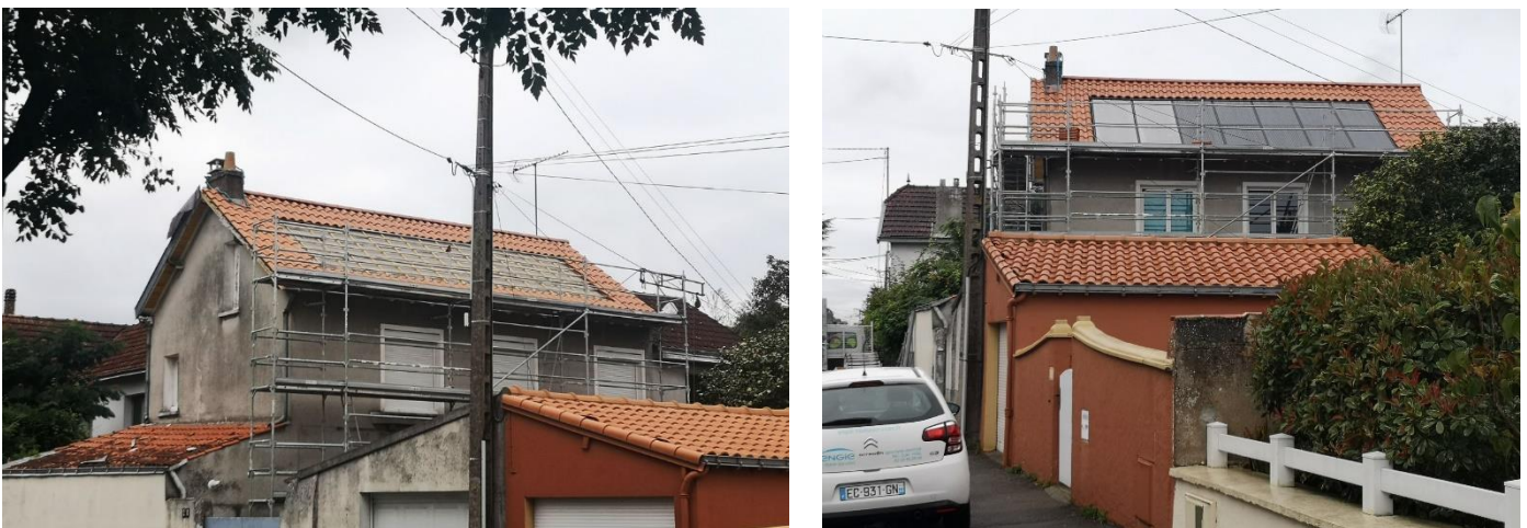
Figure 12: Pictures of the house during works (installation or R-Volt panels)
