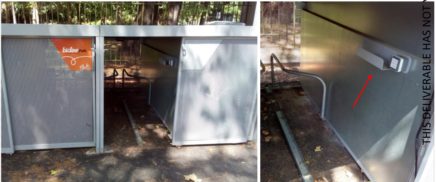
Figure 31: Individual boxes with electric socket inside
