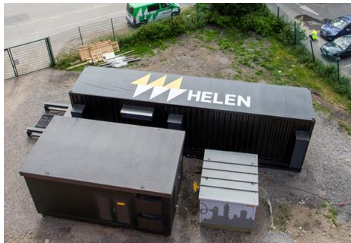
Figure 18: Battery Energy Storage System (photo: Helen Ltd.)
