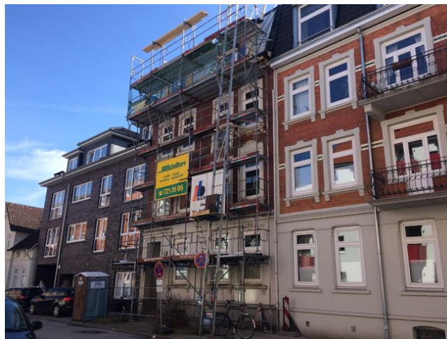
Figure 10: The retrofitting of a building at the Rektor-Ritter-Straße in Bergedorf Süd 14
